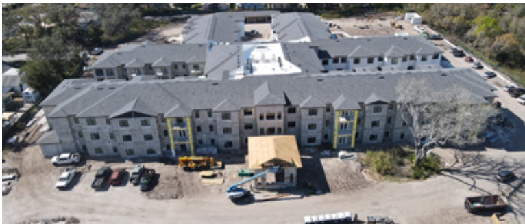
Construction progress at The Grove at Countryside
